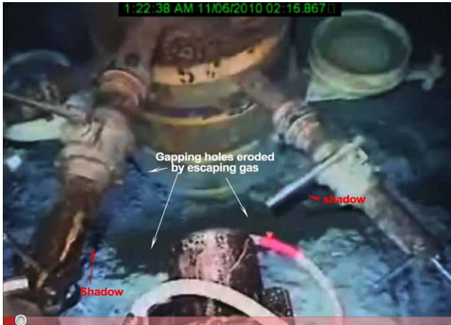
Figure : This could have been prevented: failures on the concrete seal
